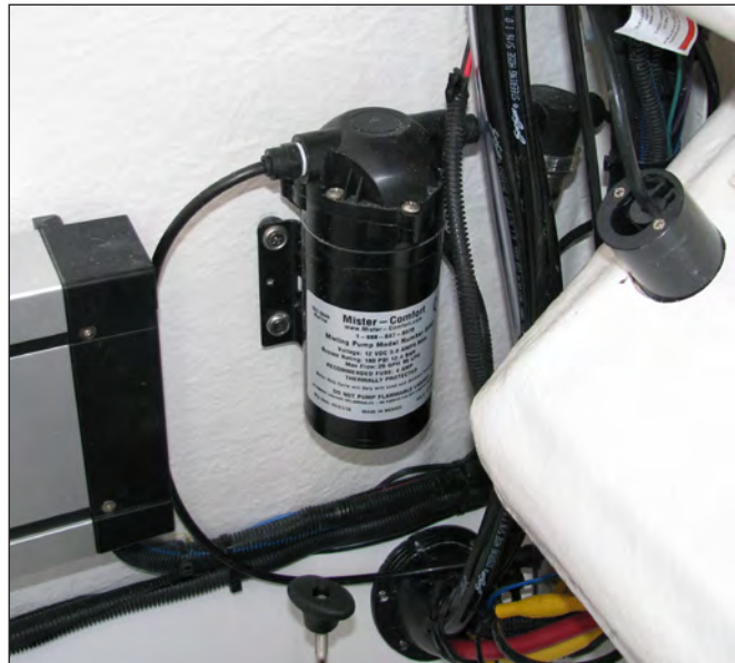
Mister Booster Pump Mounted In Center Console
