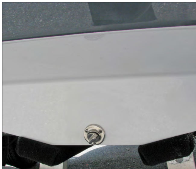
Bilge Drain Plug
