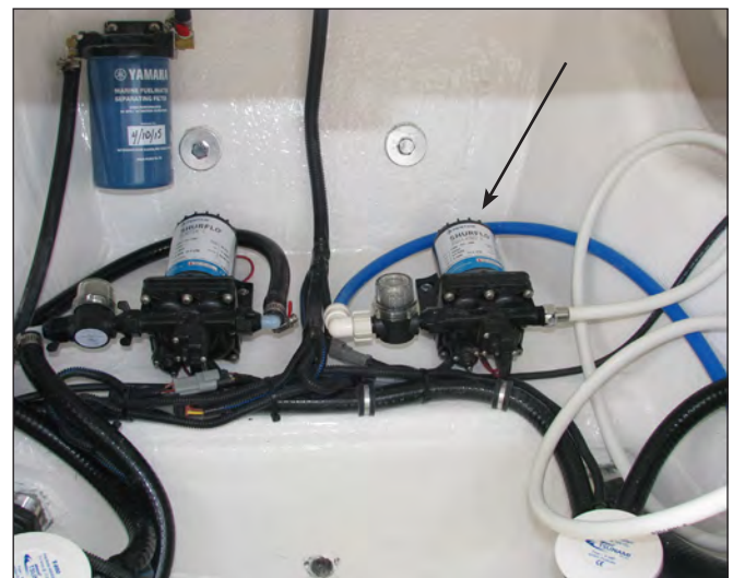
Fresh & Raw Water Pump Location In Stern Bilge
