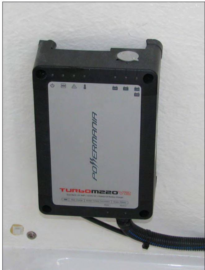
Typical Engine Battery Charger
