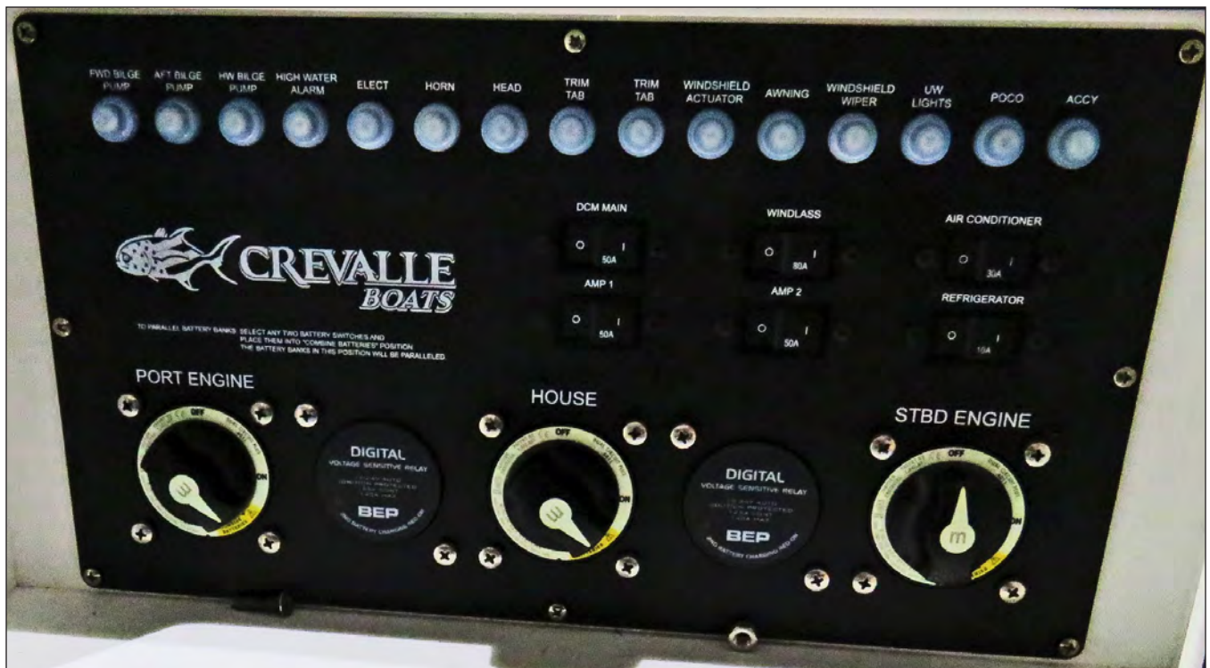
Part Engine & House Battery Switches in Parallel (COMBINED BATTERIES) Position
