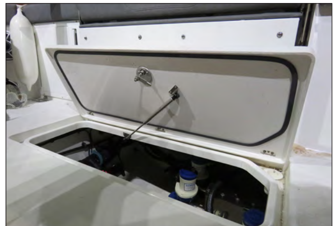
Aft Systems Compartment Hatch
