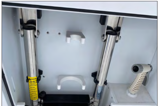
Ladder & Fire Extinguisher Compartment
